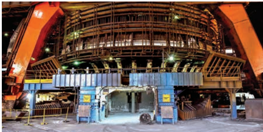
Resource-efficient blast furnaces with high productivity
