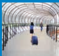
iGATE Skywalk in Bengaluru
